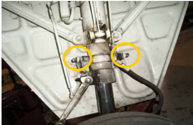
Outer gear door disconnect points
